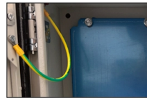
Grounding screw More aesthetically pleasing and safer
